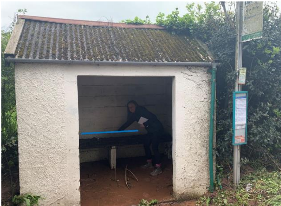
Figure 4.2 EA flood reconnaissance photo with EA staff/blue line marker highlighting the flood level reached on the bus stop at the end of Burrow, approximately Grid Reference: 307640, 089557.
