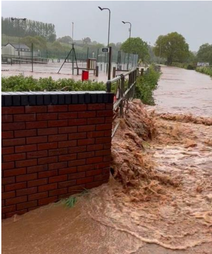
Figure 4.3 Still image taken from video post peak flows. This is looking north along Back Lane in Newton Poppleford before the Back Brook reaches the River Otter. Even following peak flows the bridge is shown as overtopping. (Resident's video submitted to EA/DCC).
